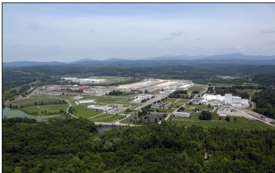
Figure 1.8. Aerial view of East Tennessee Technology Park
